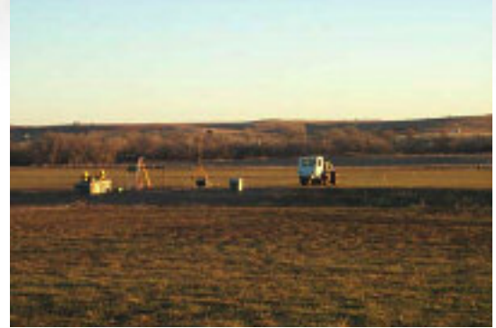
CO 2 injection well with DGPS receiver and part of the distributed seismograph.
