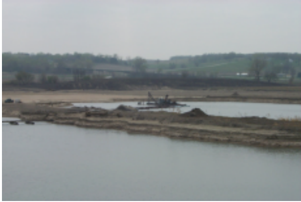
Figure 15. Sand dredge work in south end of pond.
