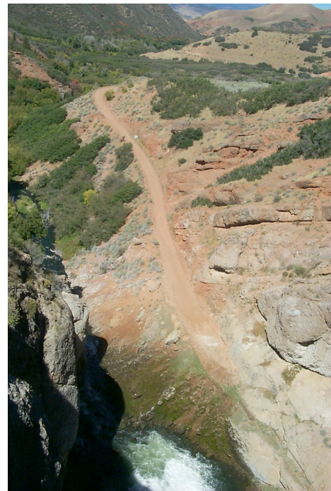
Figure 47. (right) View of the toe road from the dam crest. Dipping layers can be defined by changes in material “weatherability.”
