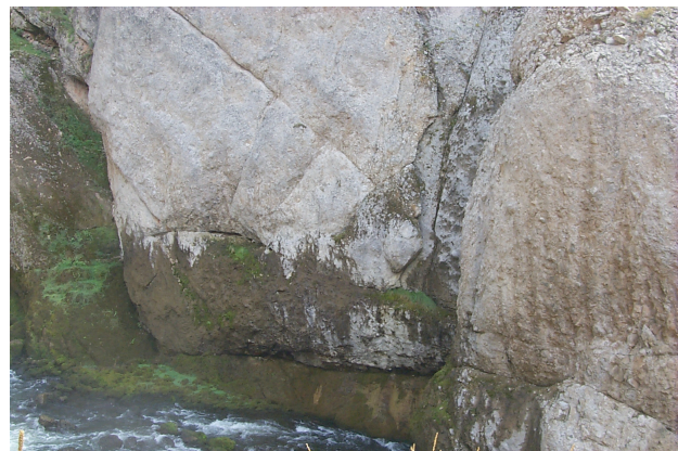
Figure 49. View looking south from toe road. Fractures can be interpreted with dips ranging from vertical to horizontal and most angles in between.
