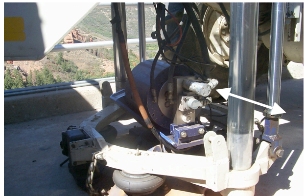
Figure 30. Vibrator mass/baseplate located on dam crest in transverse configuration.
