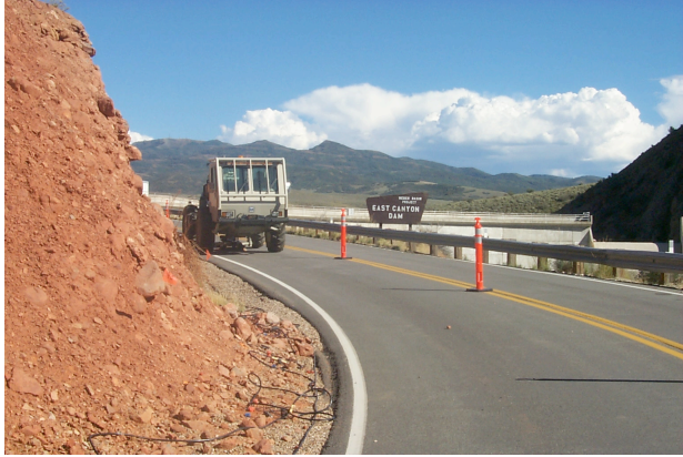
Figure 12. Vibrator setup at station downstream of dam along right abutment road. Receivers and cables in north road ditch.
