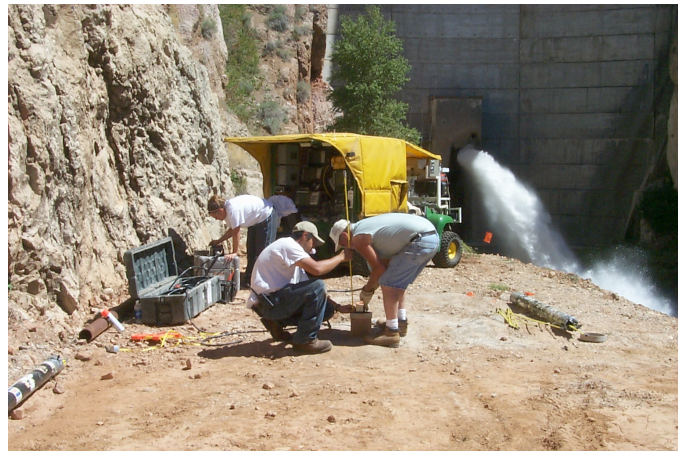
Figure 35. Toe borehole with tool being positioned and locked in place.
