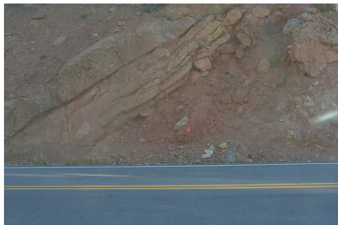
Figure 36. Abutment road with dipping bedding planes of the massive conglomerate exposed.
