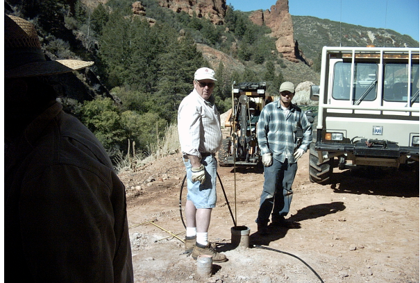
Figure 28. Cable and alignment rods protruding from the toe borehole.
