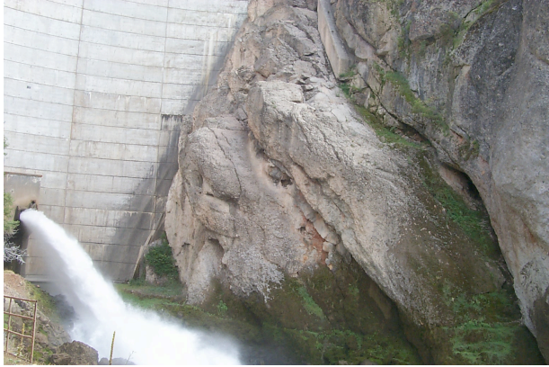
Figure 5. View of conglomerate rock, which is the foundation for the dam.
