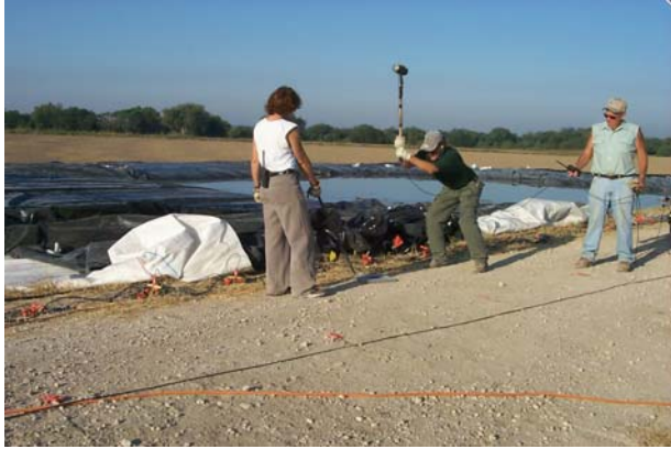
Figure 33. Compressional-wave survey during full pool.
