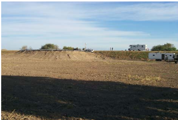
Figure 25. Pond constructed to test flood simulation interrogations.
