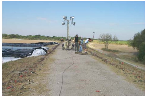
Figure 5. Shear-wave source operated along the north line at site 2 during the ponding test.
