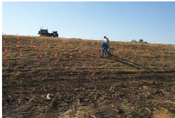
Figure 16. Source grid along north side of site 1 for through-levee study.
