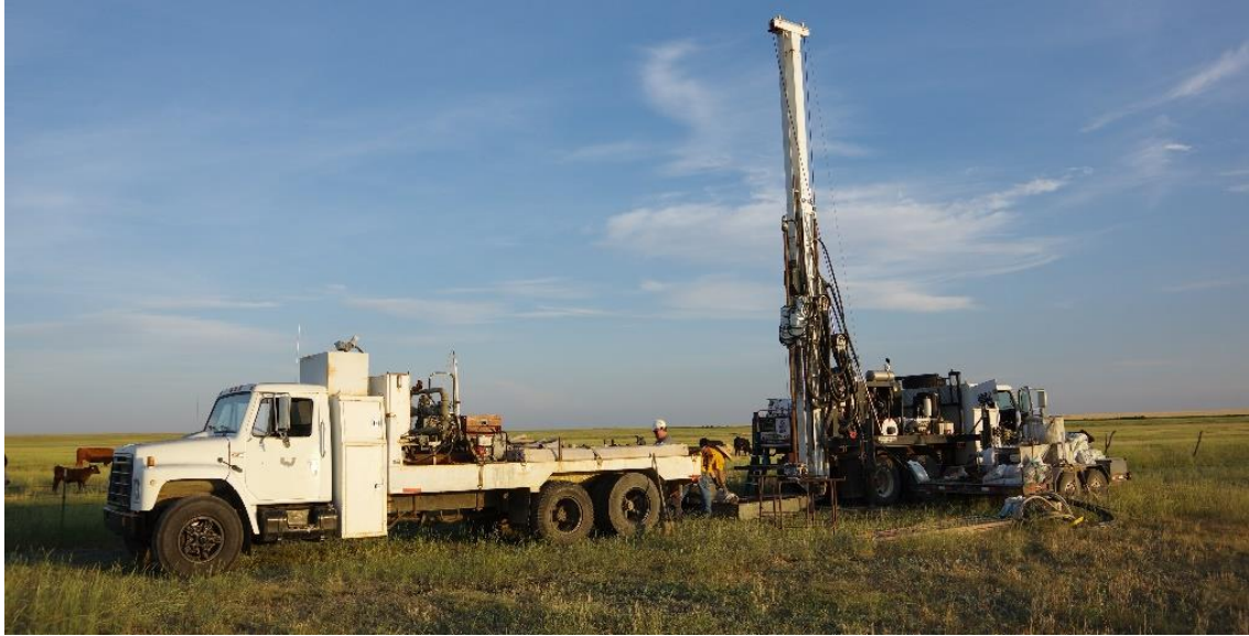
Figure 15. Kansas Geological Survey Explorations Section drill crew installing one of the three groundwater monitoring wells. (W.C. Johnson)
