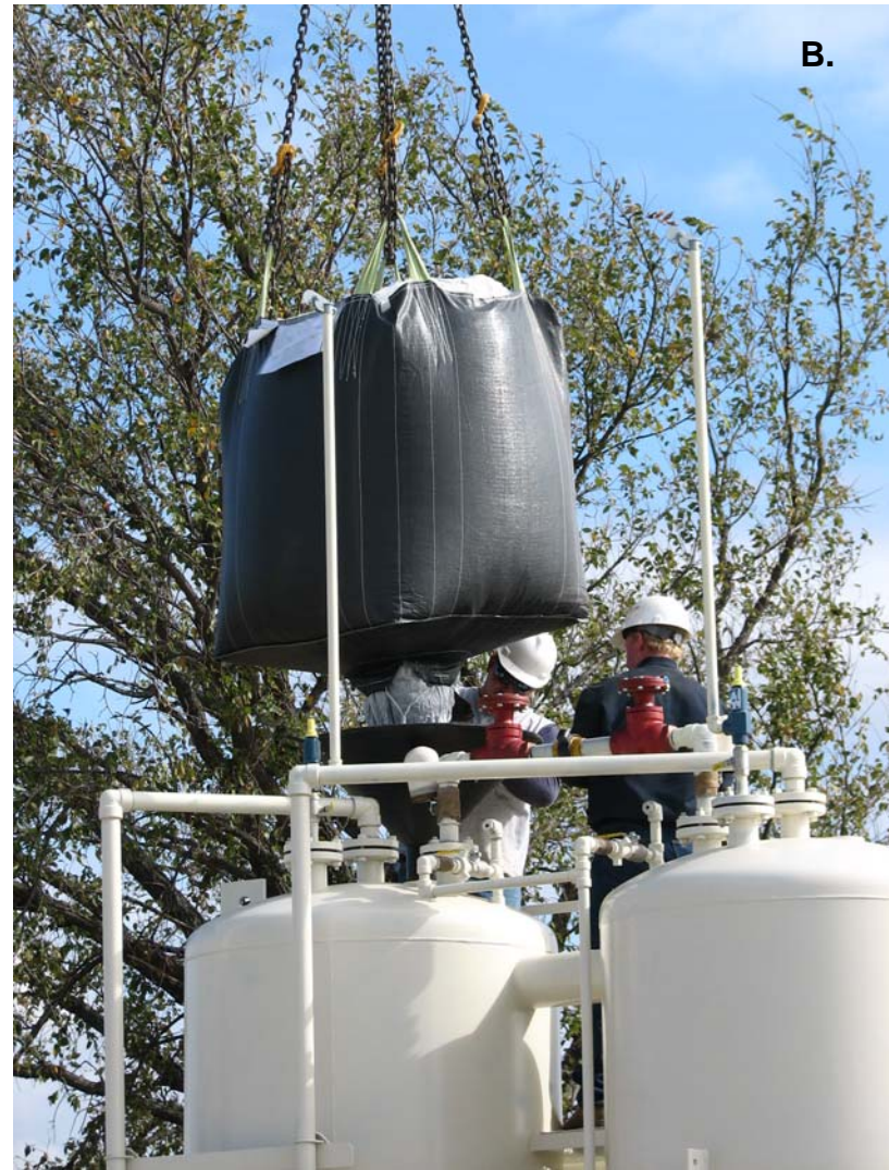
Figure 5: Pictures showing the following: A) close up of activated carbon granules, B) charging of the towers with activated carbon, and C) leveling the carbon bed after charging towers.
