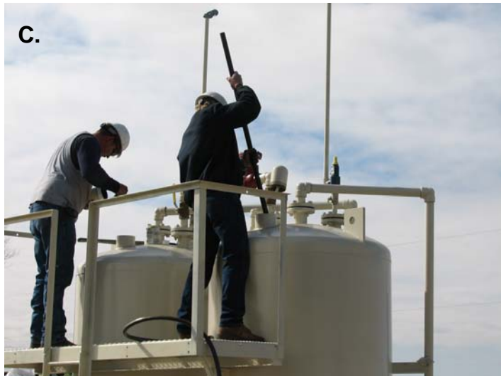
Figure 5: Pictures showing the following: A) close up of activated carbon granules, B) charging of the towers with activated carbon, and C) leveling the carbon bed after charging towers.
