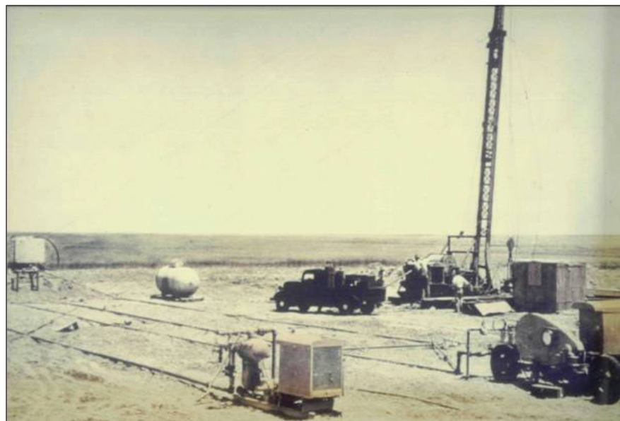
Figure 1—First experimental fracturing job conducted in 1947 by Stanolind Oil in the Hugoton gas field of southwestern Kansas utilizing “1,000 gallons of naphthenic-acid and palm-oil- (napalm-) thickened gasoline” . . . “and sand from the Arkansas River” (from Montgomery and Smith, 2010, p. 2).
